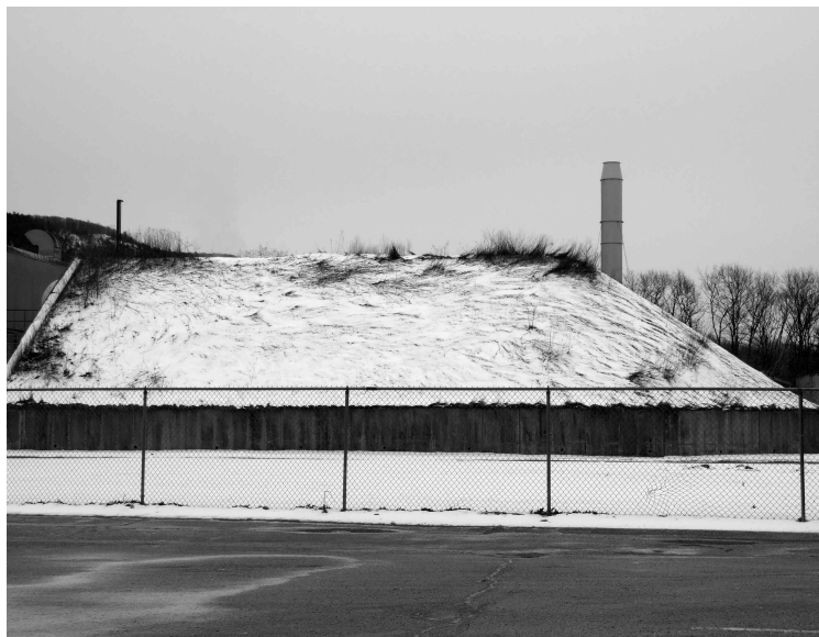
A large earth-covered structure attached to the plant shields the area in which packaged syringes are sterilized by ebeam.
